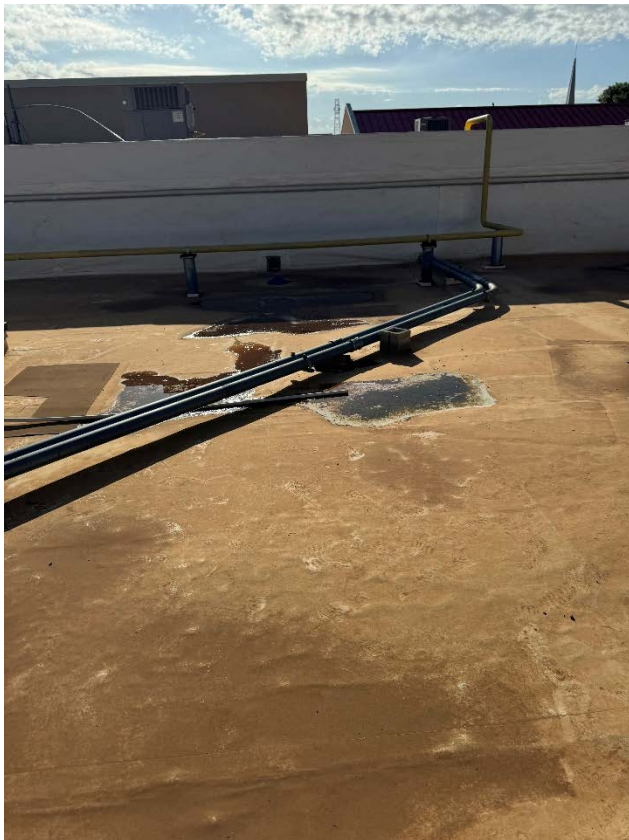
Figure 11 –Roof Ponding
