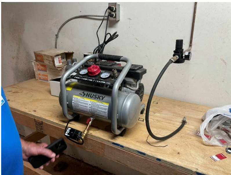
Figure 47 - Existing Heating System Control Air Compressor
