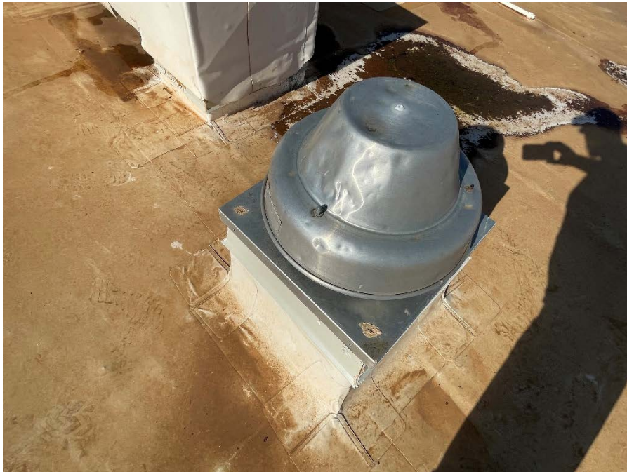
Figure 30 - Hail Damaged Exhaust Fan
