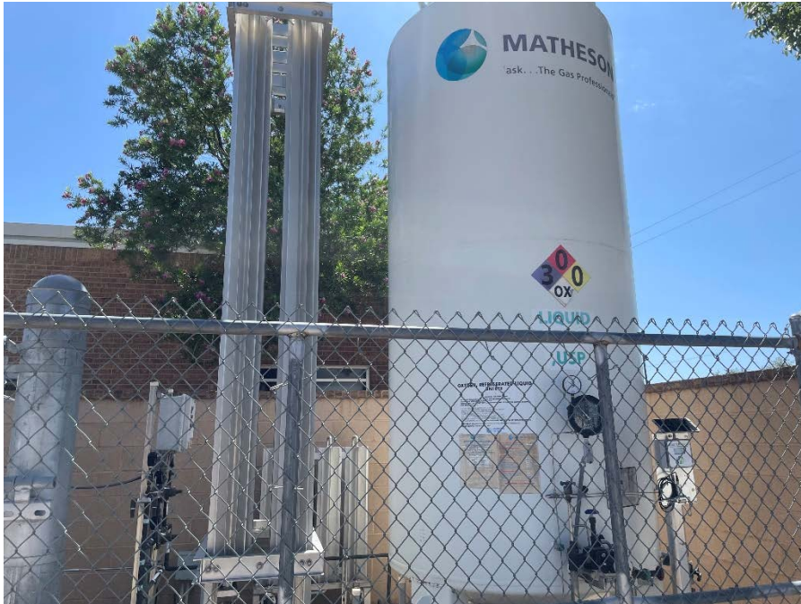
Figure 36 - Bulk Oxygen Supply System
