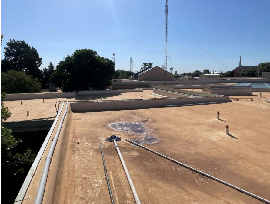
Figure 33 - Example of Roof Sag
