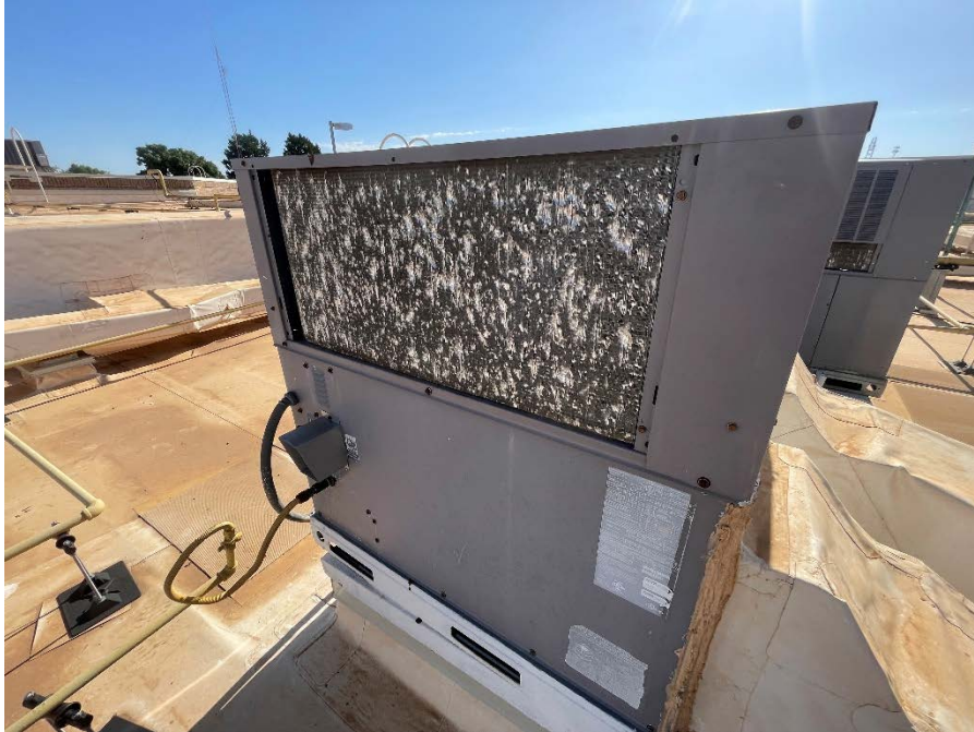
Figure 45 - Hail Damaged RTU Condenser Coil Fins
