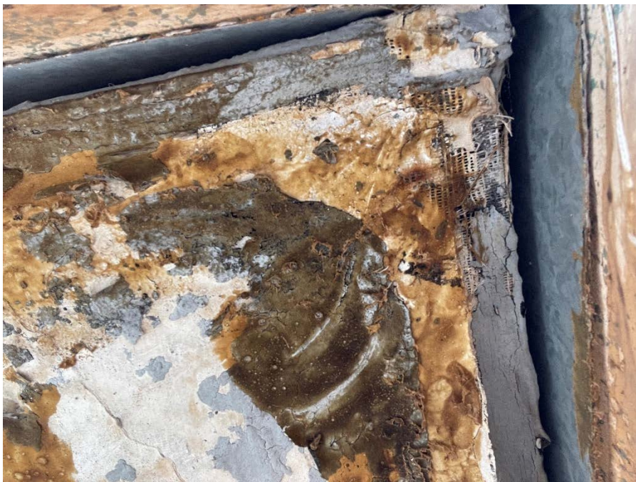
Figure 21 - Example of Exterior Ductwork Degradation, bottom view of ductwork
