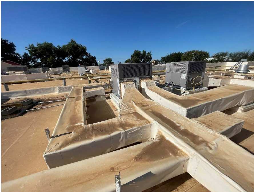
Figure 19 - Example of RTU's with Exterior Routed Ductwork
