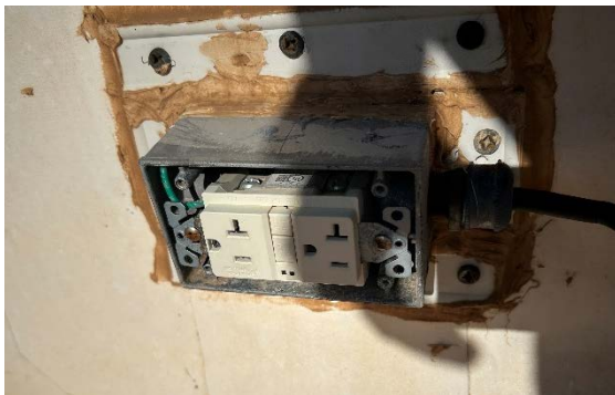
Figure 48 – Electrical Box Missing Cover
