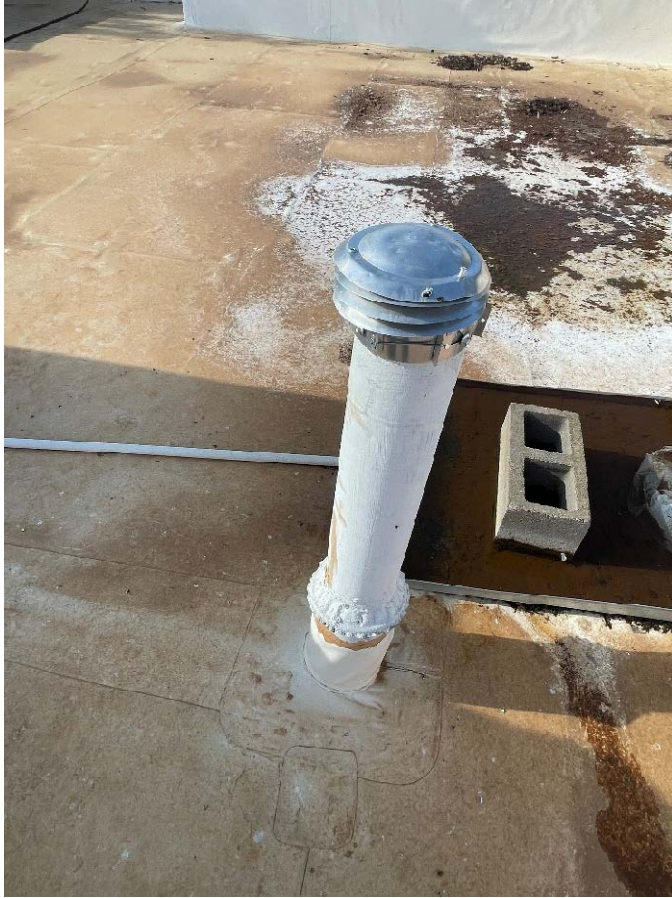
Figure 29 - Hail Damaged Flue Vent Termination
