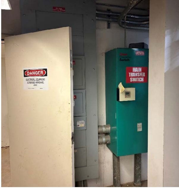
Figure 45 – Main Transfer Switch Blocked by Column
