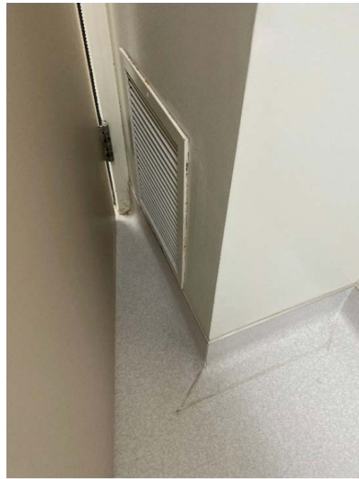
Figure 39 - Low Return in Operating Room, rust showing on edges
