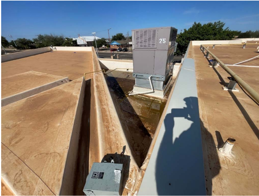
Figure 35 - Roof Area with Poor Drainage
