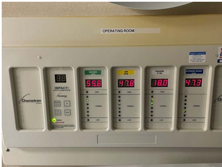
Figure 40 - Example of Operation Room Medical Gas Alarm Panel
