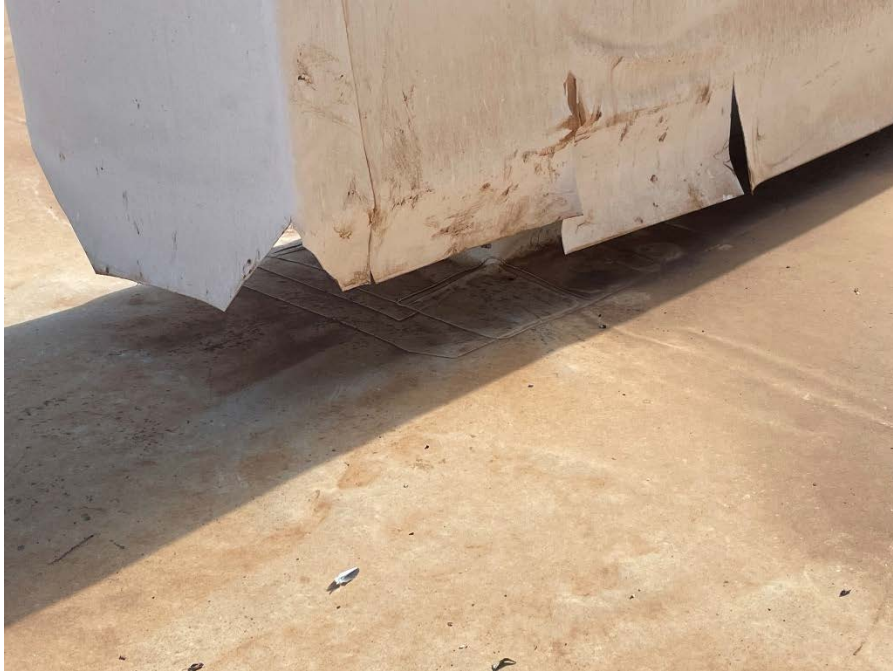
Figure 20 - Example of Exterior Ductwork Degradation, visible portion
