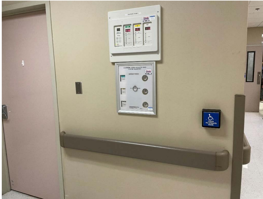
Figure 39 - Example of Medical Gas Zone Valve and Alarm Panels
