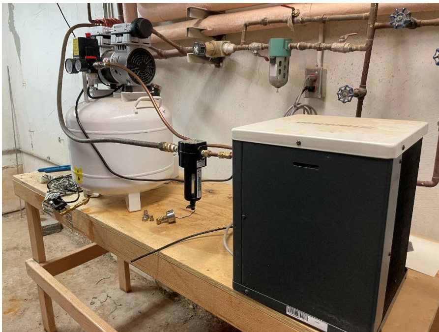
Figure 38 - Existing Medical Compressed Air System
