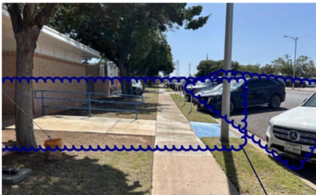
Figure 9 – Non-Conforming Ramp and Parking
