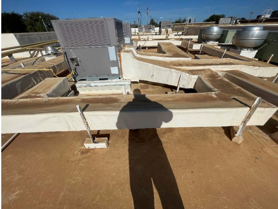
Figure 22 - Example of No Outside Air Intakes on RTU's
