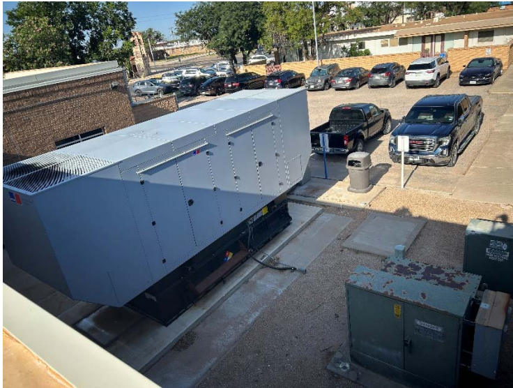
Figure 63 – Generator and Utility Transformer
