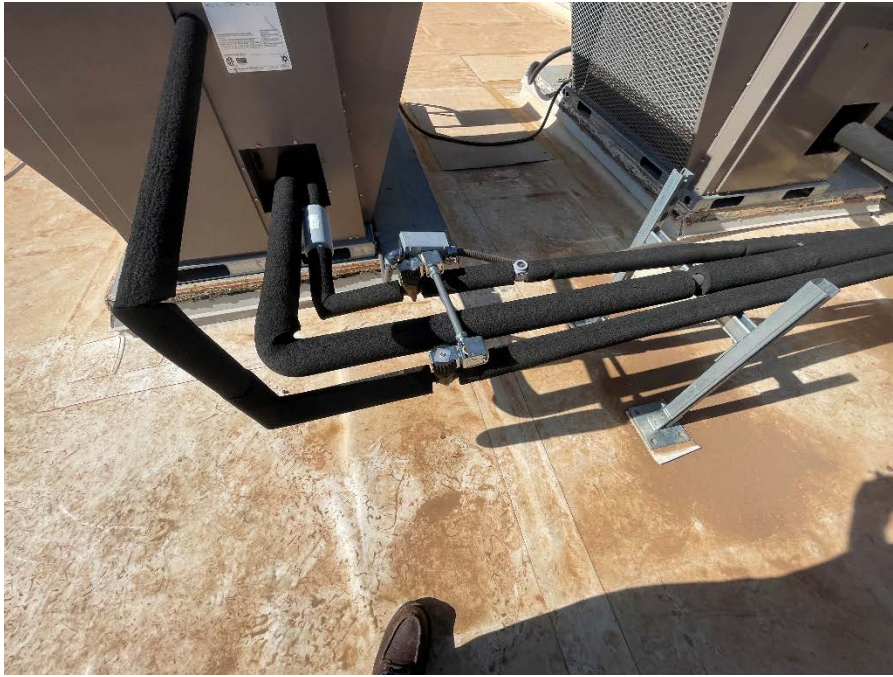
Figure 42 - Existing Refrigerant Roof Piping Insulation
