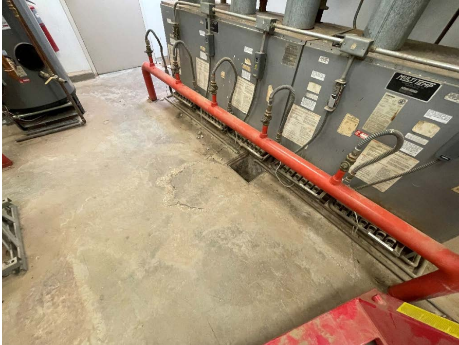
Figure 31 - Existing Natural-Gas Fired Heating Water Boilers
