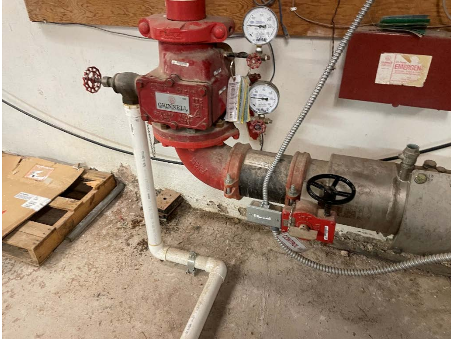
Figure 42 - Existing Fire Riser Valve and Backflow Preventer
