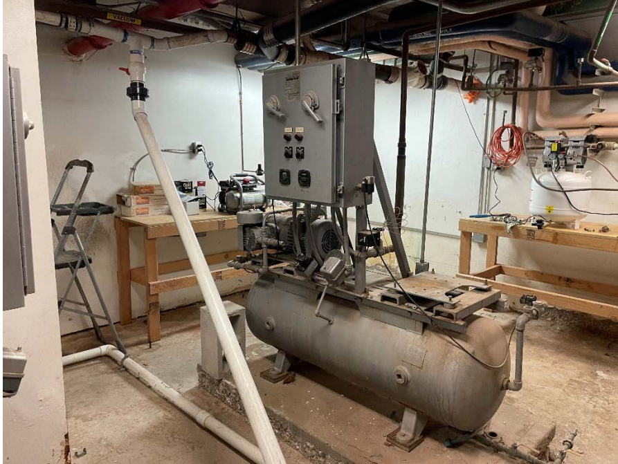
Figure 37 - Existing Medical Vacuum System
