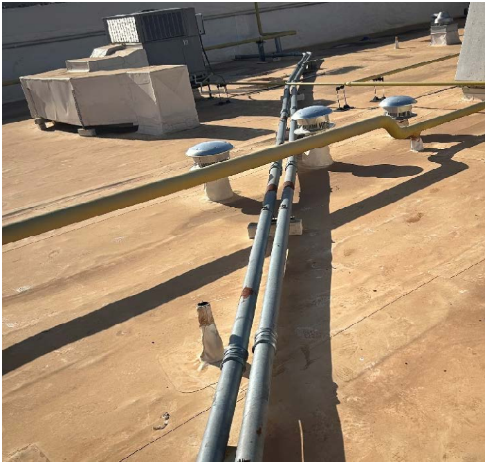
Figure 69 – Roof Conduit
