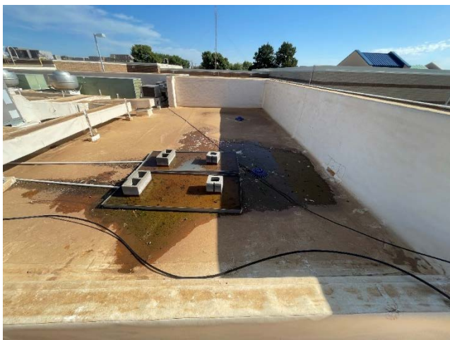
Figure 23 - Existing Condensate Evaporation Pans
