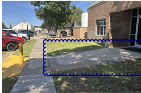
Figure 8 – South Entrance to Rehab Too Steep
