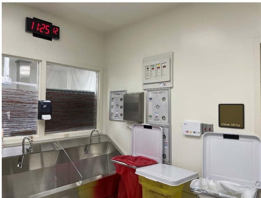
Figure 41 - Questionable Access to Medical Zone Valve Assemblies
