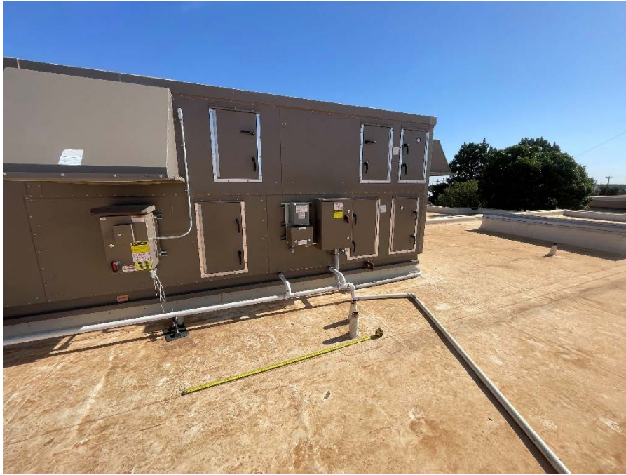
Figure 24 - Plumbing Vents Closer than 25'-0 to RTU
