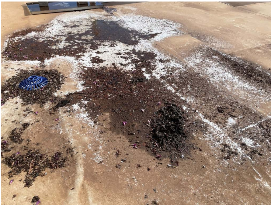
Figure 34 - Example of Roof Sag, Debris, and Severe Ponding
