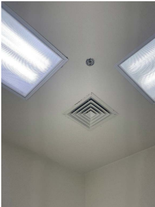
Figure 26 - Ceiling Supply in Operating Room, rust showing on the edges
