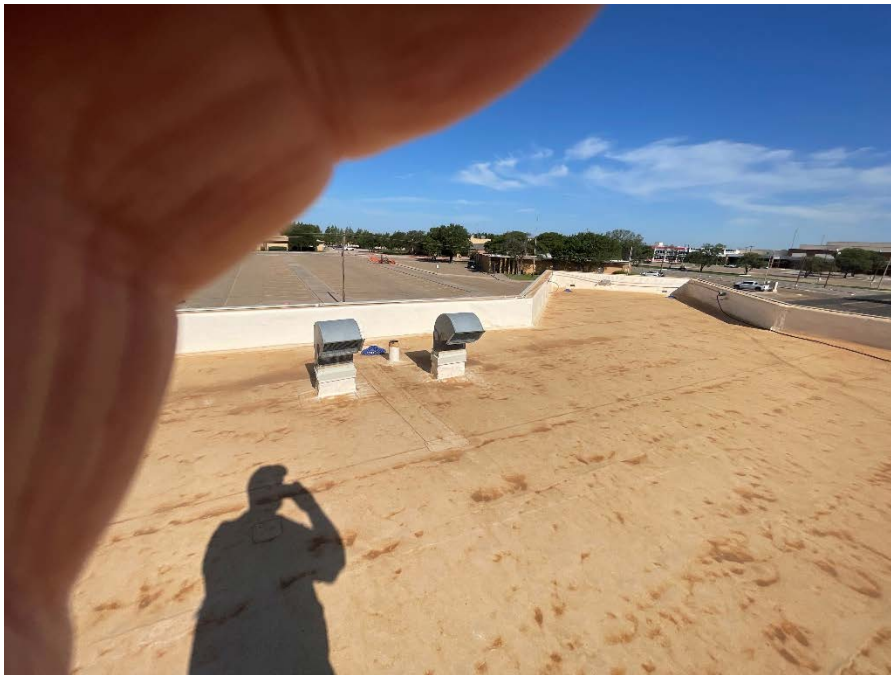
Figure 28 - Existing Goosenecks on Hospital Roof
